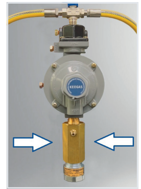
Installation example of SENTRY GS excess flow valves for LPG installations
